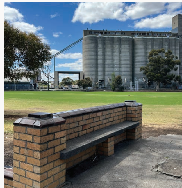
Heritage silos backdrop to the east of the site
