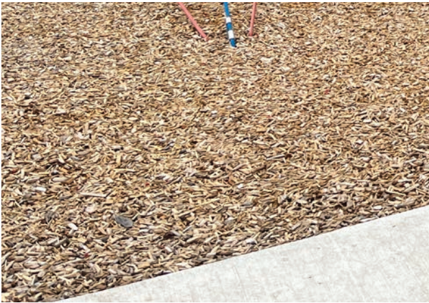
Concrete & mulch softfall
