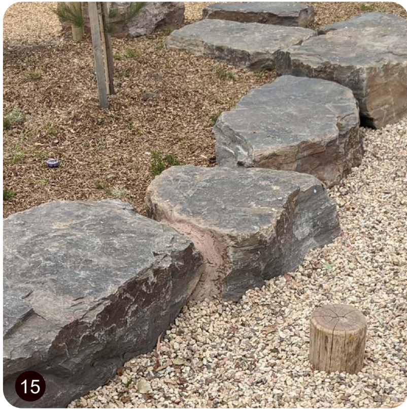
15 Mudstone Boulders Pink Sedimentary derived Mudstone with flat tops. 500-800 x 600-1000mm Heights Vary. Max. 550mm above FSL. Gaps between boulders to be mortared.
