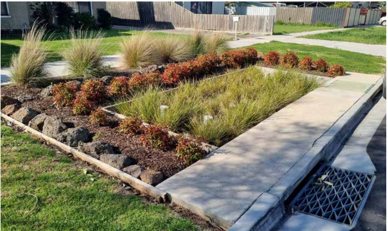
Raingarden at front 4 Essex St, Sunshine North. Jamie Comley, Environmental Consulting
